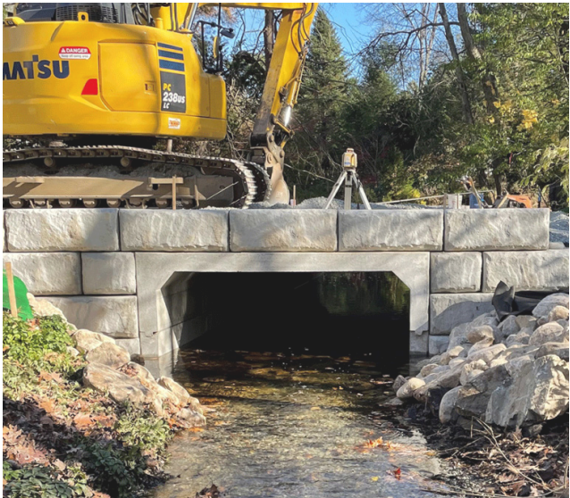
Fg 17. Weston Culvert Replacement (© Wright-Pierce)
