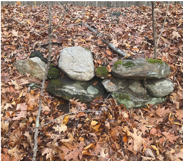
Fg 7. Culvert CU139 - Outlet Fully Obstructed
