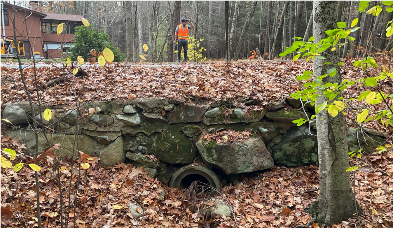
Fig 1. Nitsch Team Assessing Culverts Across the Town
