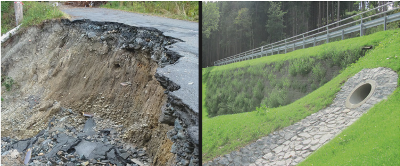
Fg 15. Embankment Repair (© Geosynthetica)
