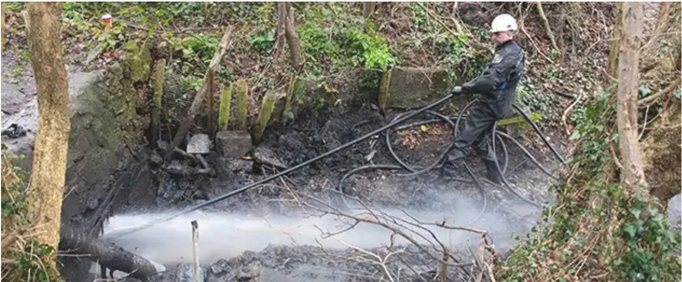
Fg 14. Culvert Cleaning & Vegetation Removal (© HCL)
