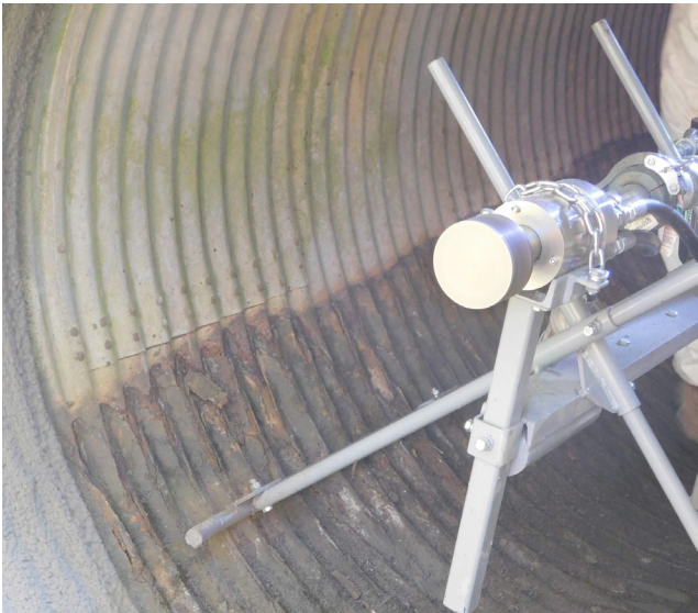
Fg 16. Spin Cast Lining (© National Plant Services)
